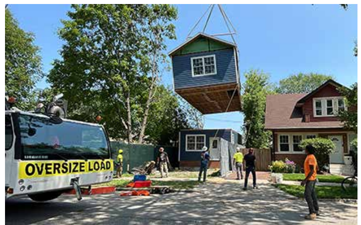
For the 8th house, both floors were moved from the Evanston campus last summer to Brown Ave. and hoisted into place by a giant crane. The interior of the house was to be completed later in 2023, and the affordable home was to be ready for a family to move in next year.
